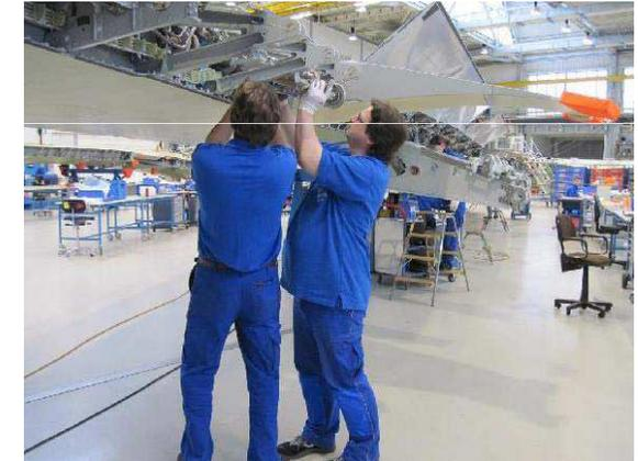
Einbau Hydraulik Pylon Cross over
